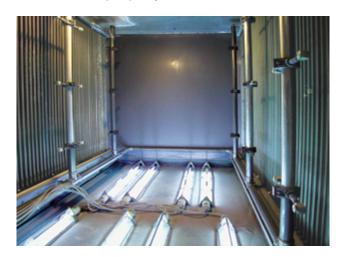
and hardness in order to prepare the proper spatial distribution of the UV-STYLO modules. In **air conditioning systems**, the 'UV-STYLO-E is directly applicable in the **tanks for collecting the water used for humidification system (cooling)**. The excess of such water, after being sprayed against the evaporative panels, percolates in tanks and, then, is recycled. The units are placed considering a UV dose of 1 watt of rated power (0.33 W UV-C) for every 1.5 dm3 water.
